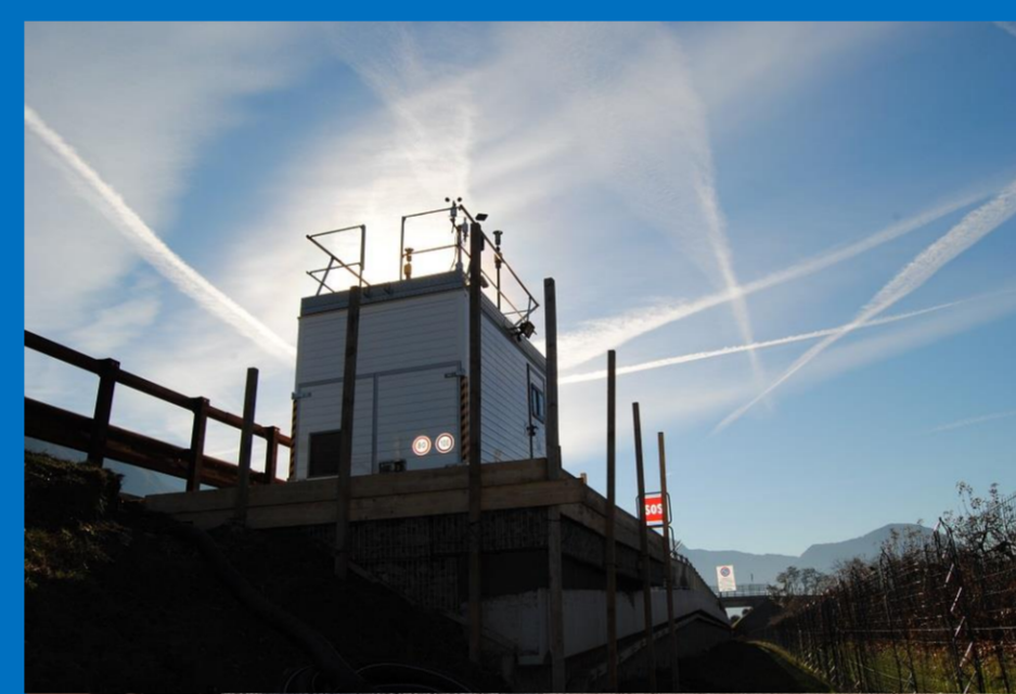
Air quality station installed along the Brenner highway.
