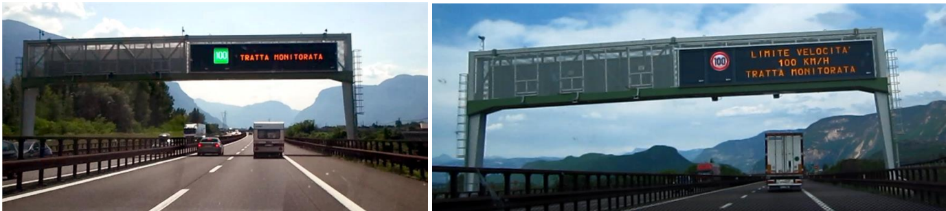
Figure 4 – VSL triggered by poor air quality conditions in different testing conditions: suggested speed limit (on the left) and mandatory speed limit (on the right) .
