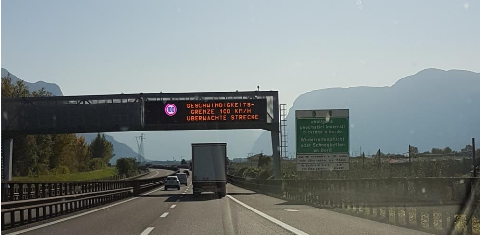
Figure 2 – Message displayed on the “entry VMS” during test sessions in the BLEC-AQ test stretch.
